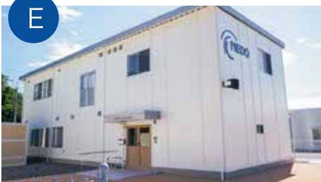
Common Use Building
